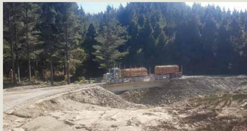
The moveable bridge was built by Bridge It NZ. It is an 18m x 4m steel beam bridge with timber deck capable of holding a full load required for forestry truck and trailer units and heavy machinery.
